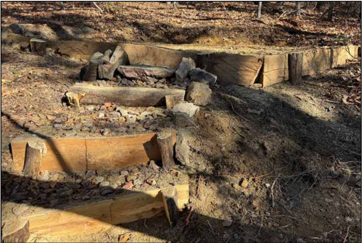
A completed tent pad with stairs and cribbing.
