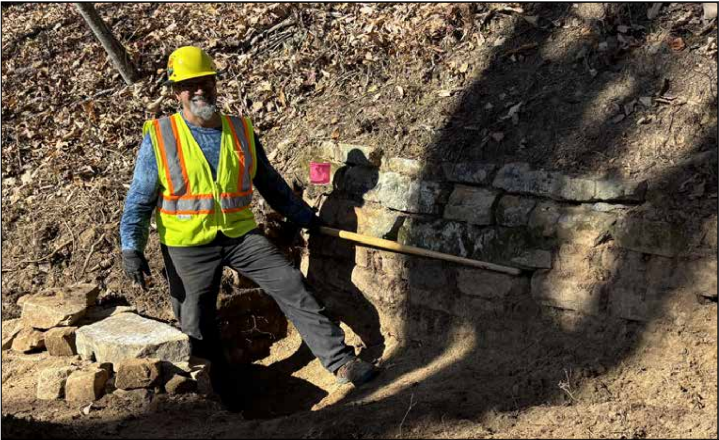
In addition to mechanized work, shovels and picks were used too. Dario Izquierdo uses a tool handle to show the depth of collected sediment removed to clear a culvert. The original rock work is exposed.
