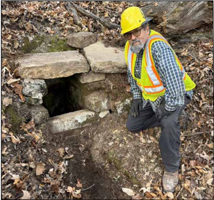
Dario Izquierdo next to the stone work for a reclaimed drain. Many of these have been covered with sediment and debris. 10 Culverts and were completely recovered and 66 drains were constructed or reconstructed.
