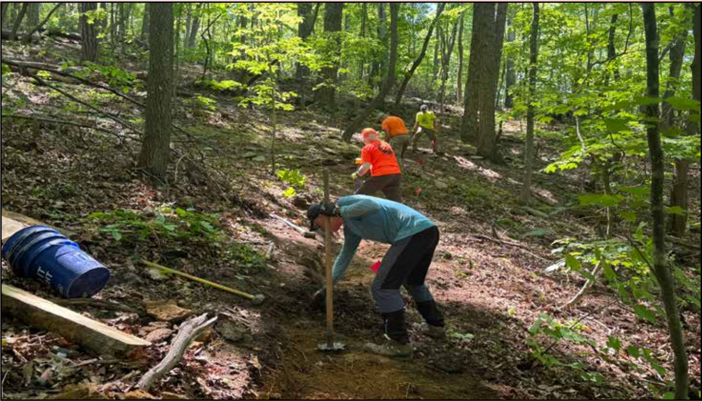
Digging the long steep trail to the Catawba water source.
