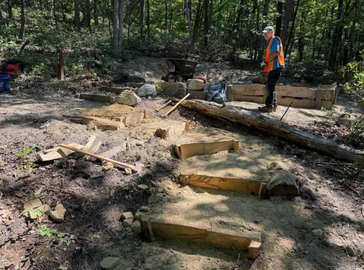
Mike Vaughn completing stair work on the last Catawba shelter tent pad showing stair work and cribbing with large locust logs. Each of the large, durable, logs was split and carried to the tent site.
