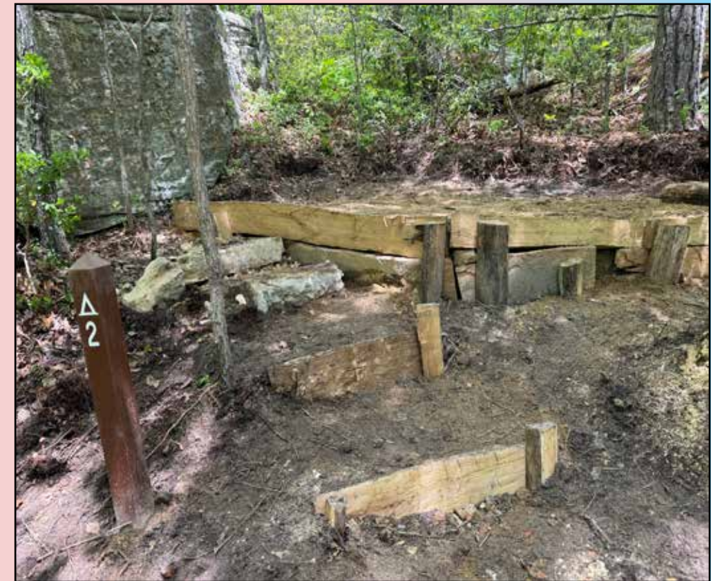
Tent pad 2 showing the cribbing, steps and signage typical of each pad.
