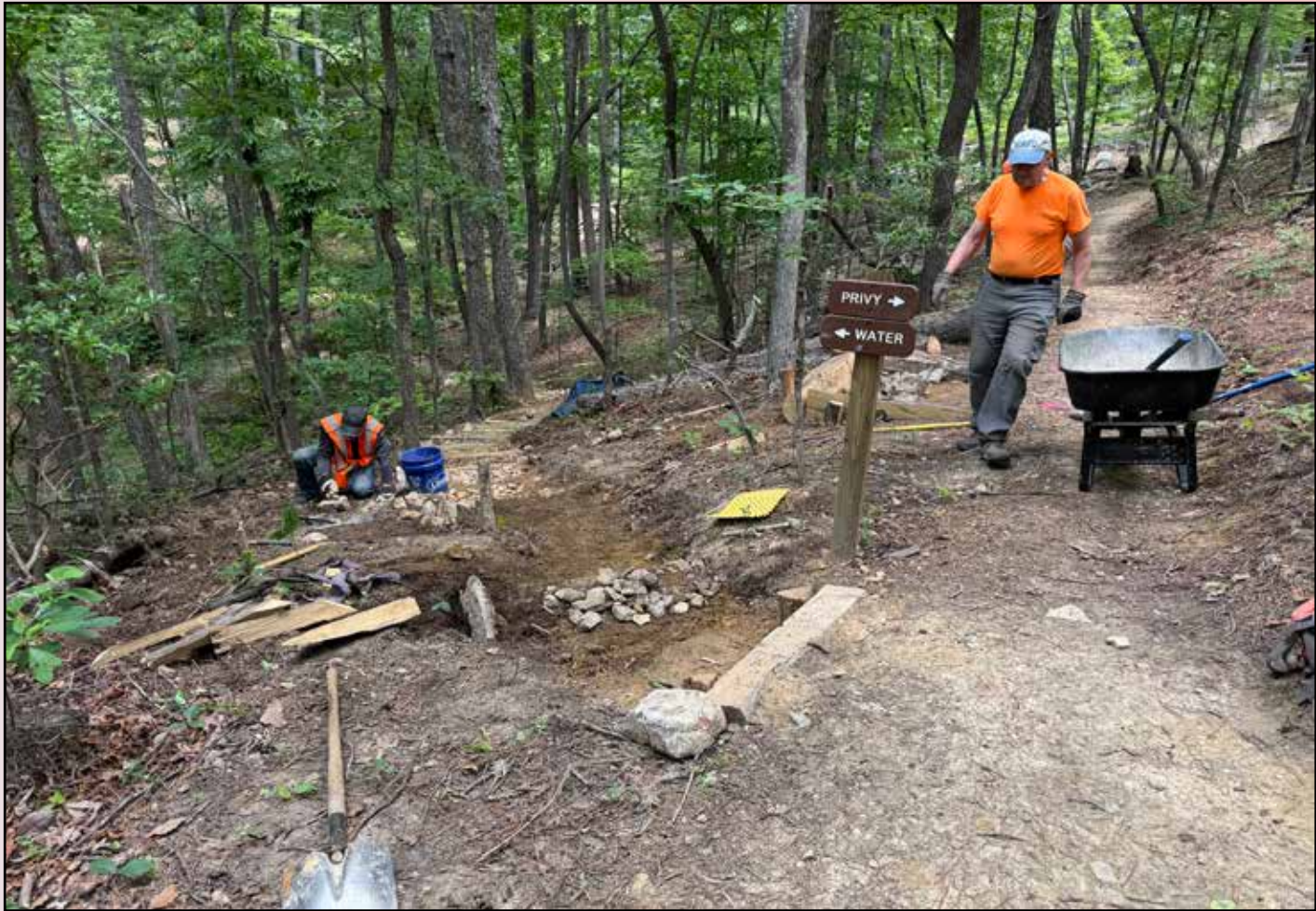
Catawba tent pad water source trail showing step construction and newly installed signs.
