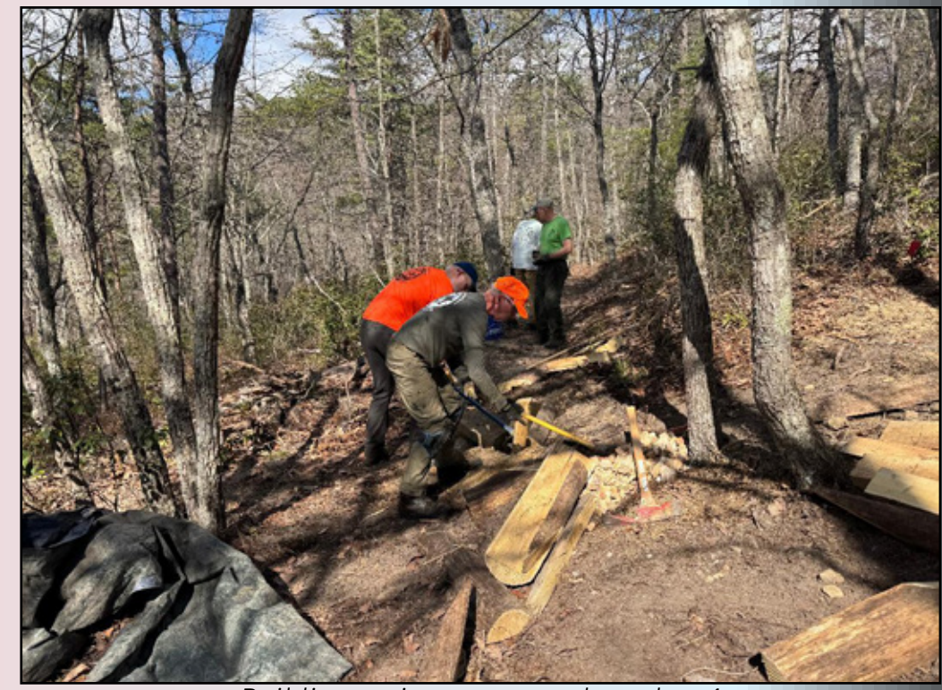
Building stairs to tent pad number 4.
