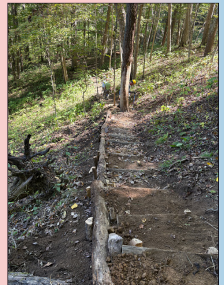
Log steps constructed near Angels Rest on October 1st.
