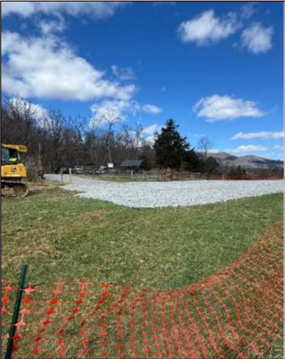
Parking lot construction at the new Andy Layne trailhead. Photo credit to ridgerunner David Nova.
