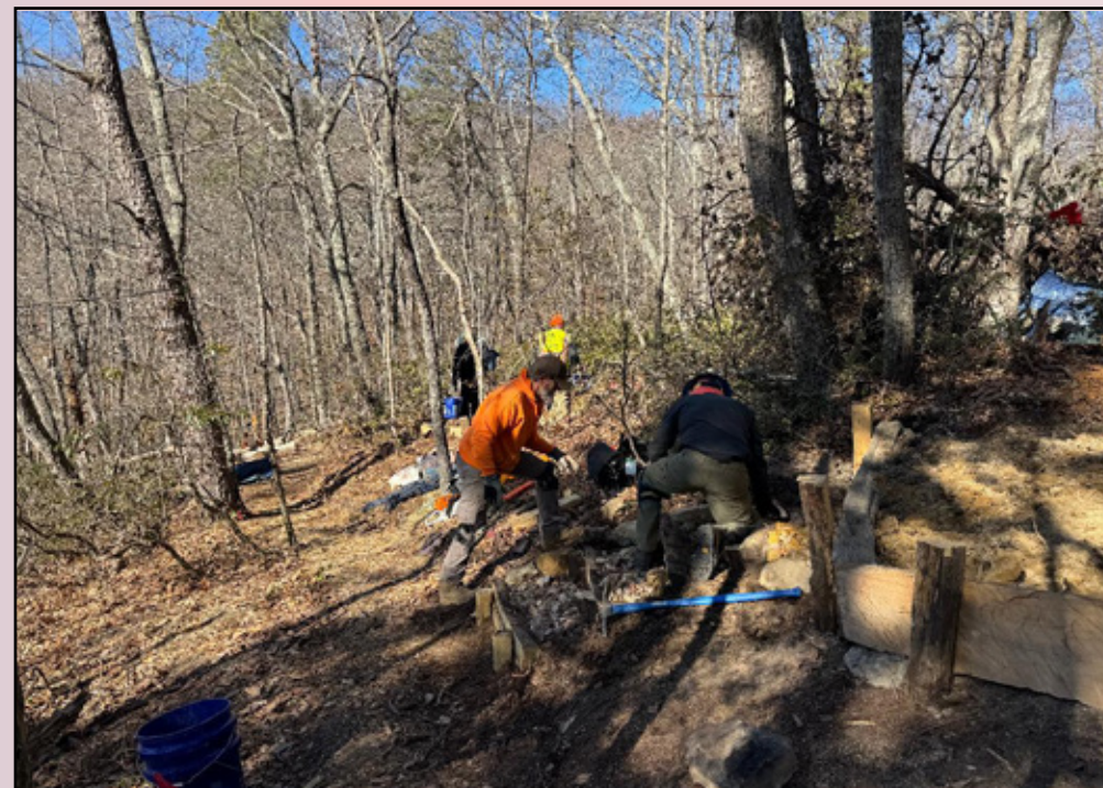
Cribbing a tent pad.
