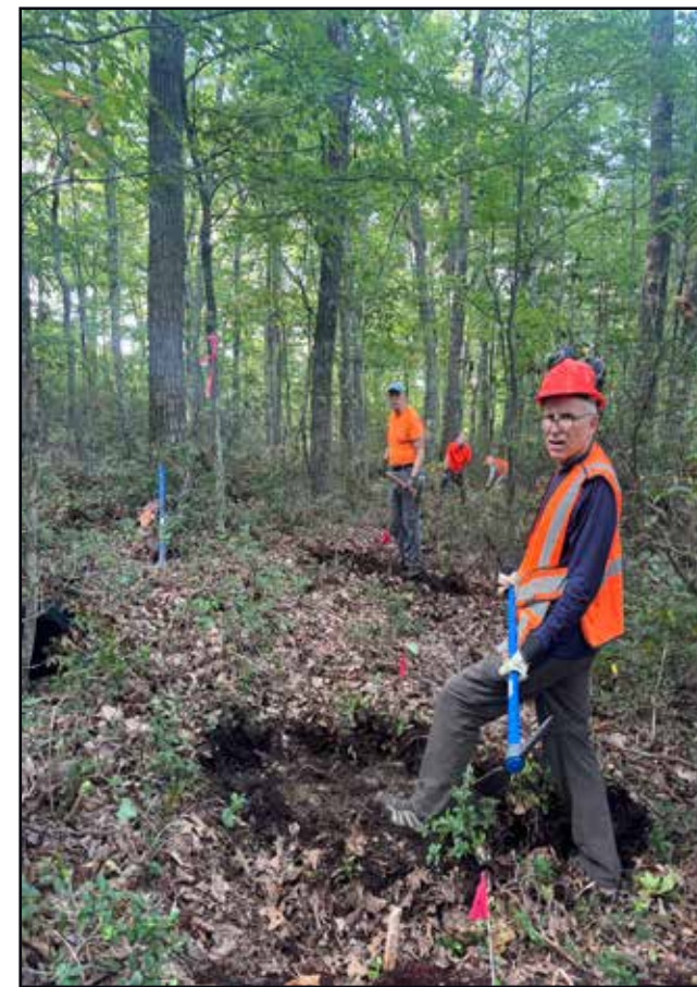
extending the Catawba shelter trail relocation from the work started by the Konnarock Crew.
