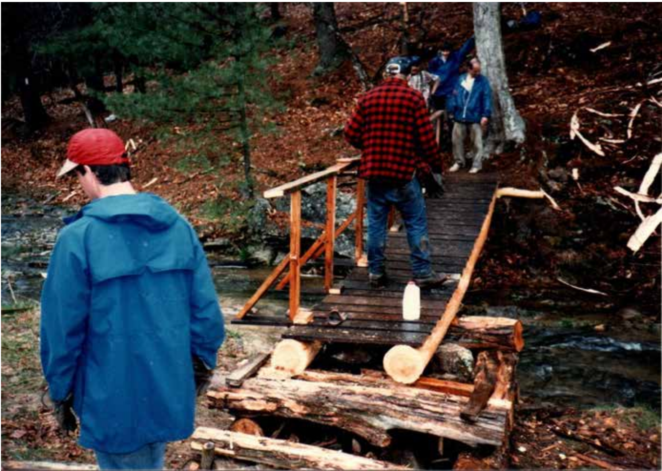
Andy Layne Trail Construction
