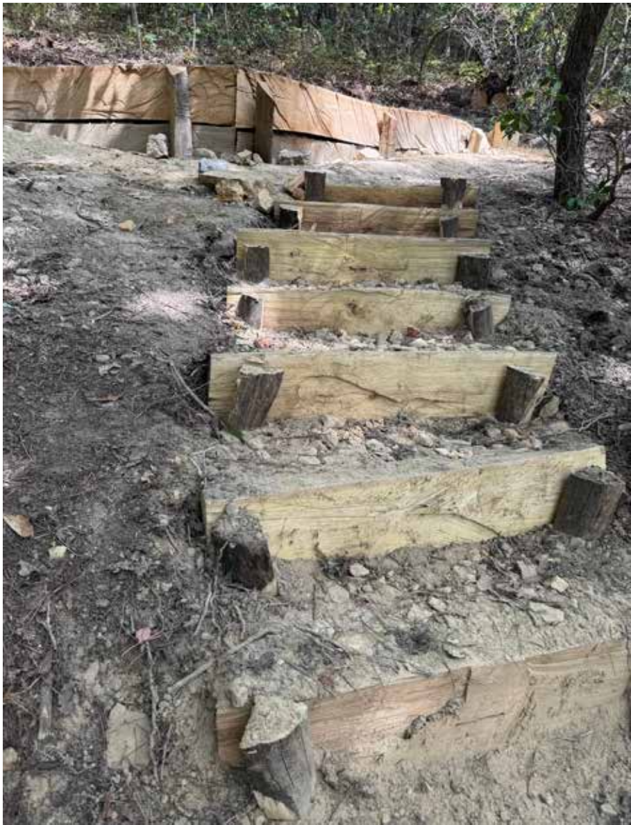
Completed tent pad access steps at Catawba Mountain
