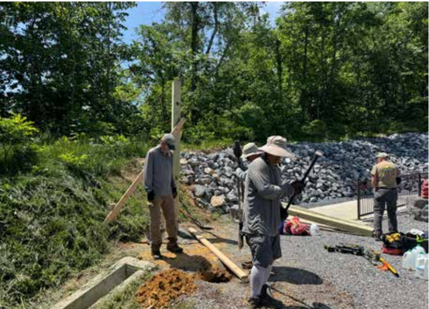
Preparing post holes for the new kiosk location
