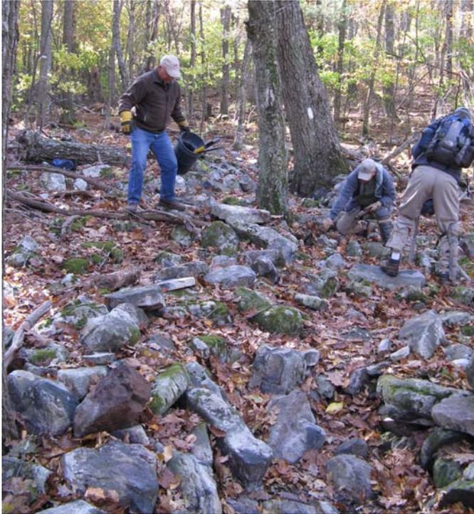
Instead of having to find and move rocks to construct steps, this project was to rearrange the jumble of rocks to provide a better path. Rock bars, leather gloves and sledge hammers aided the hands that hefted, flipped and rearranged the rocks. The effort stoked the internal furnaces, and layers of fleece, pile, flannel and wool were taken off and set aside.
